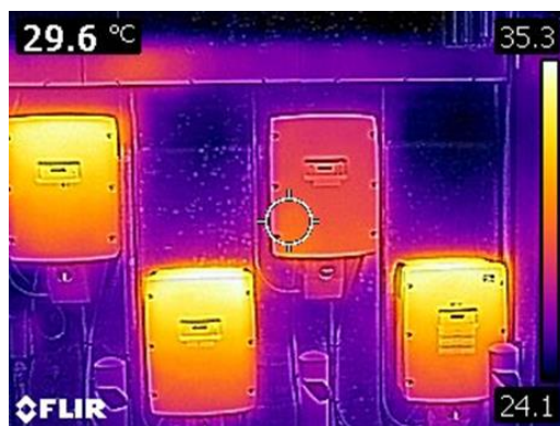
Figure 16. An anomaly, and we found all the inverters operating but the top right inverter was having a minor issue which would trip off line for a couple of minutes then run for a few minutes then shut down. This was an underperforming unit but all light indicators stated it was operating.
