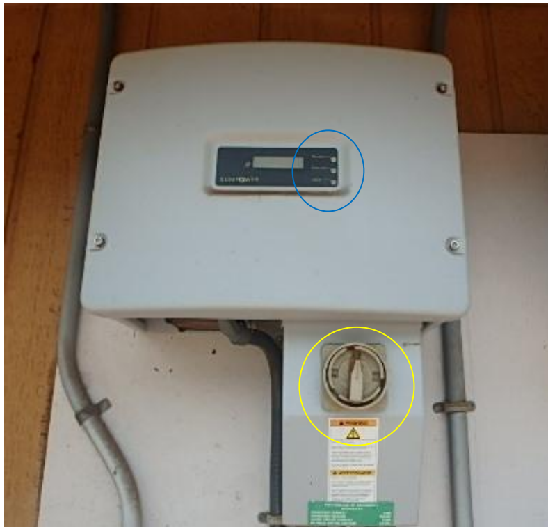
Figure 1 turn the handle to the off position and you will see the lights blink then go dark – handle is circled in yellow the lights circled in green
