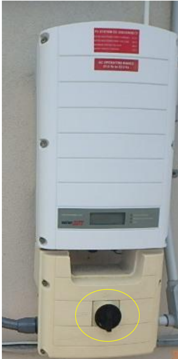
Figure 2 Turn the handle to the off-position handle is circled in yellow
