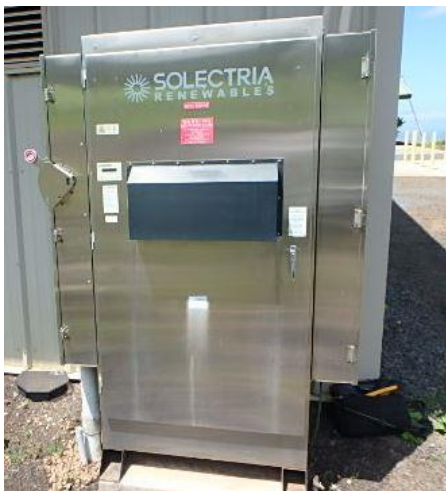
Figure 9 Solectria inverters the handles are on the left and right side – Same thing shut the DC side down first then the AC side
