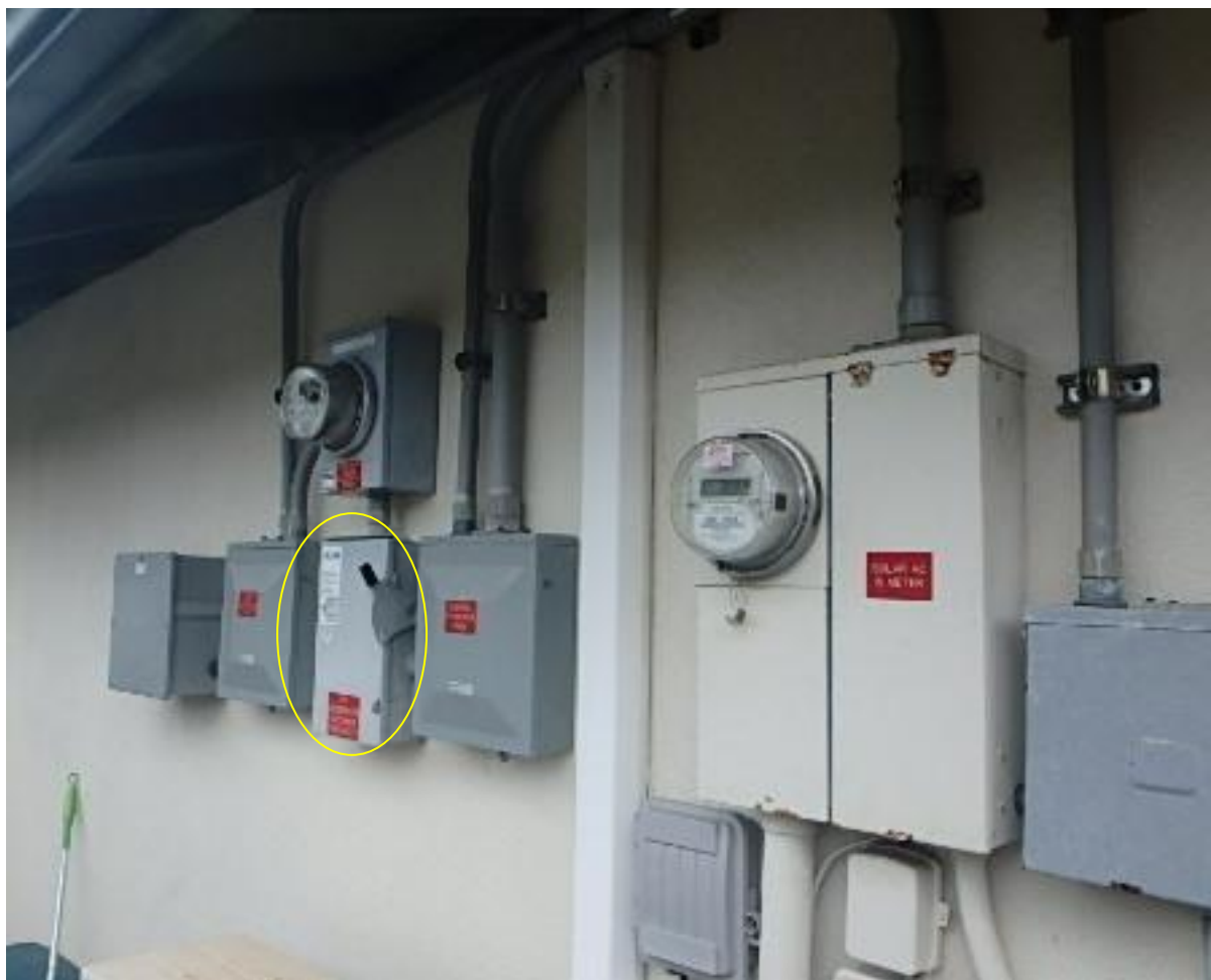
Figure 3 you will see a unit with a handle it is called a knife edge handle- this is circled in yellow now you want to make sure it is for your PV system as it should be labeled and state.
